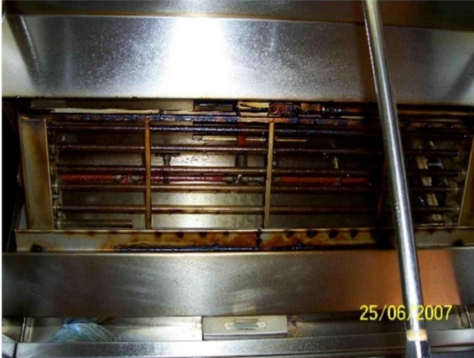
Photo of Canopy showing the state of the tubes
